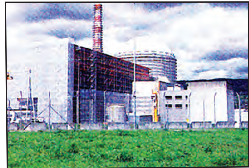
Fig. 3.16 : Nuclear power station , Kalpakkam
