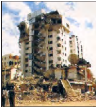
Fig. 3.3a: Destruction caused by an Earthquake in Gujarat
