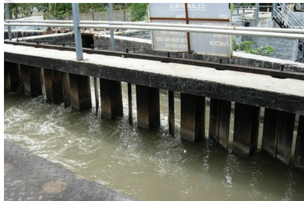
Fig. 18.4 Grit and sand removal tank
